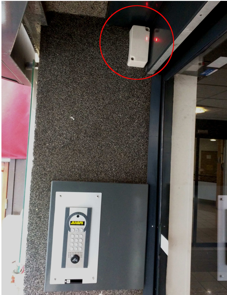
Figure 2: 3G block of an Intratone intercom
